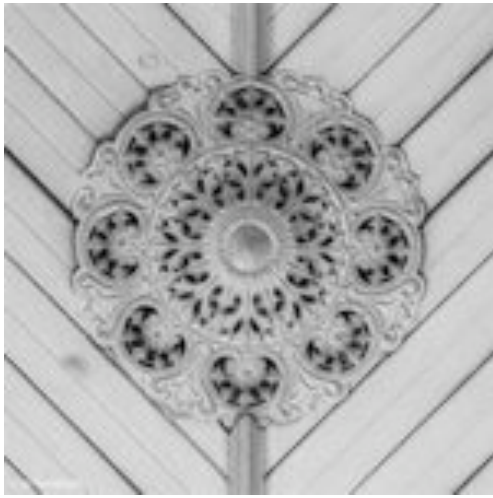
St Paul's ceiling
